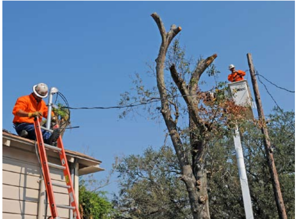
Line mechanics repair a service drop, bringing yet another customer back online.
