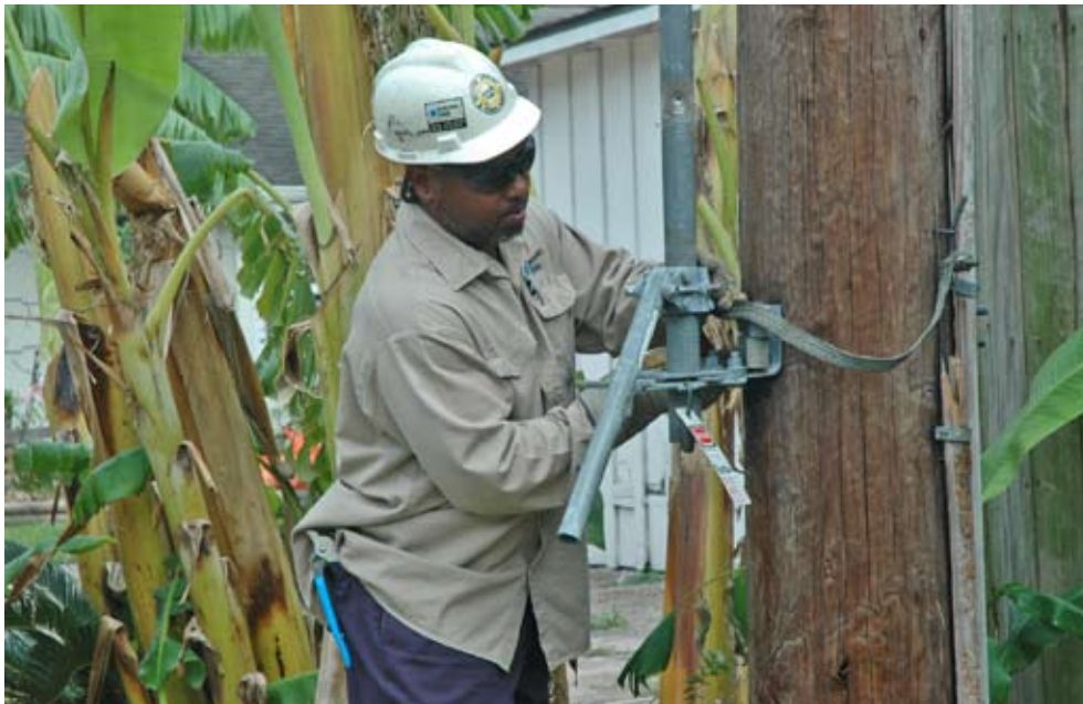
Melvin Hicks, head line mechanic, repairs a pole top switch.
