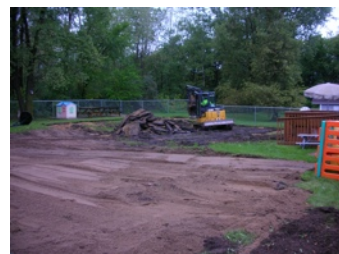
NPL clearing area for the new playground
